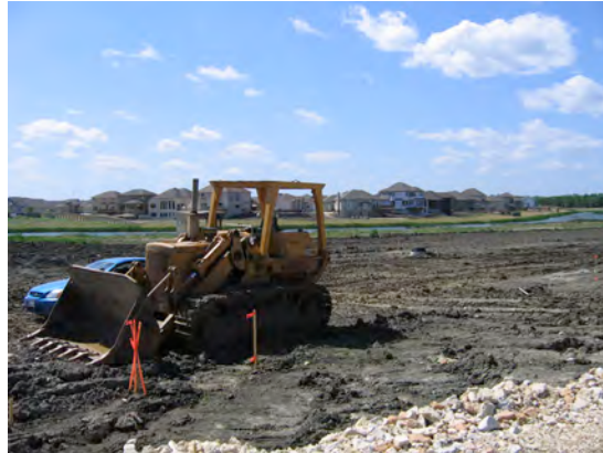
Figure 2: Land Preparation for New Suburban Development, South Winnipeg
